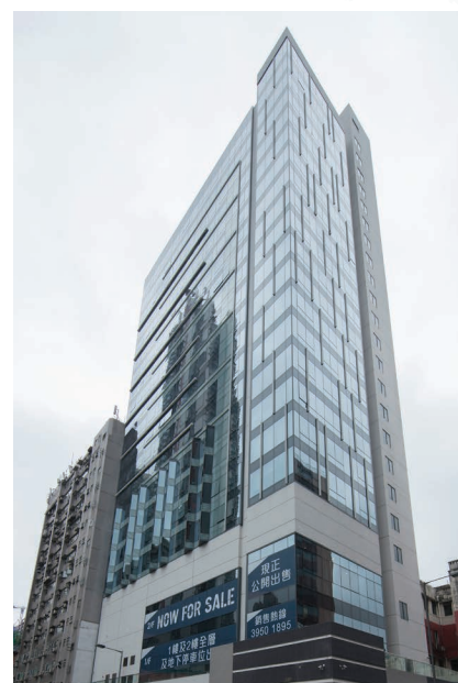
Hong Kong KHORA (Modernised industrial building)
